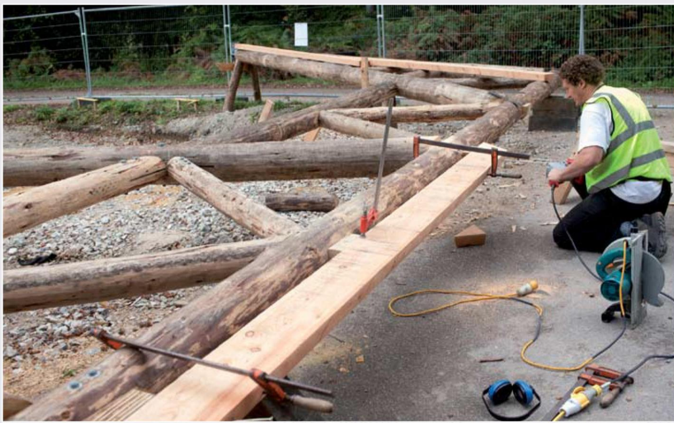
Build up at the truss top chord (backing rafter and packers installed)
