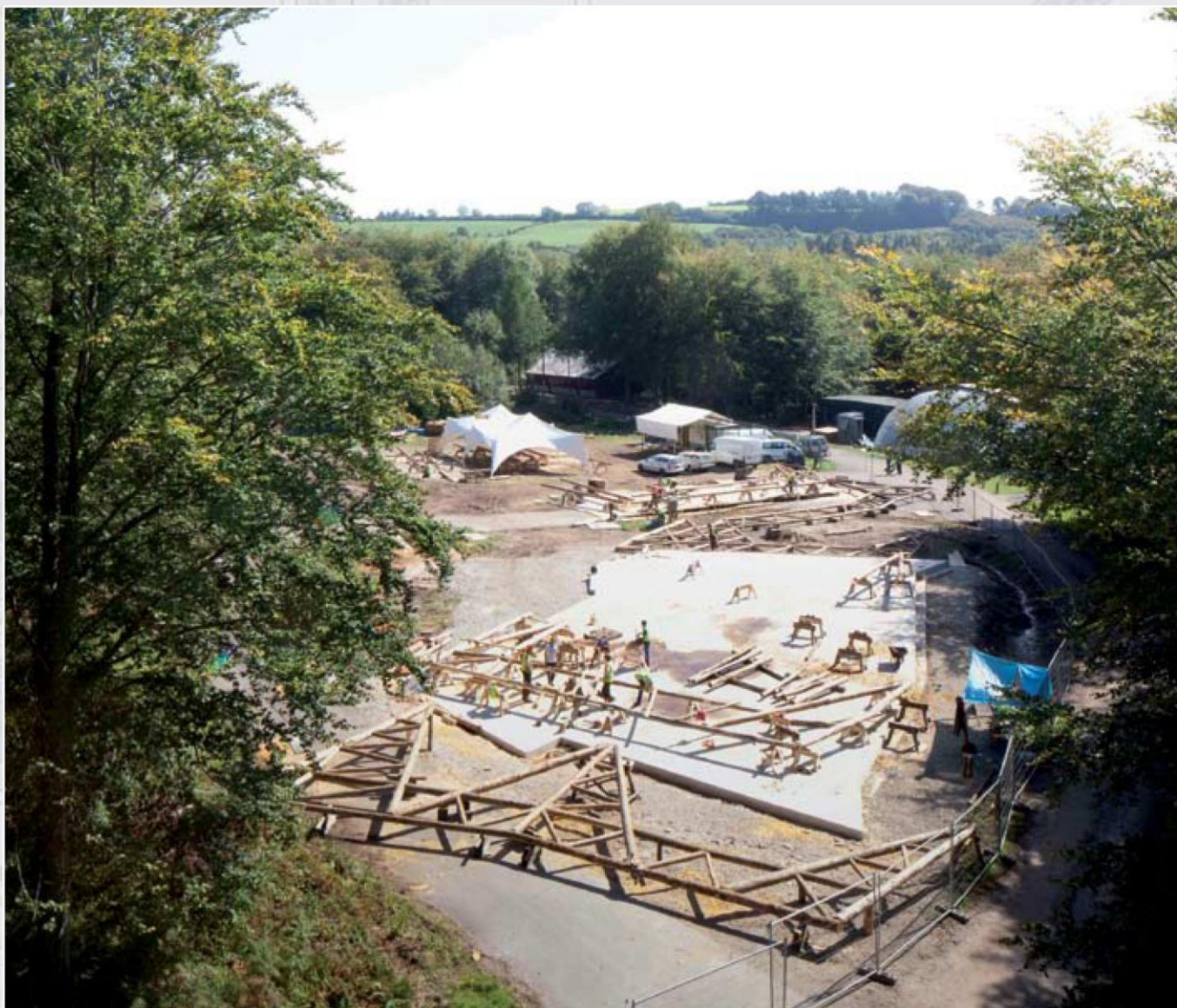
Aerial view of the initial stages of construction
