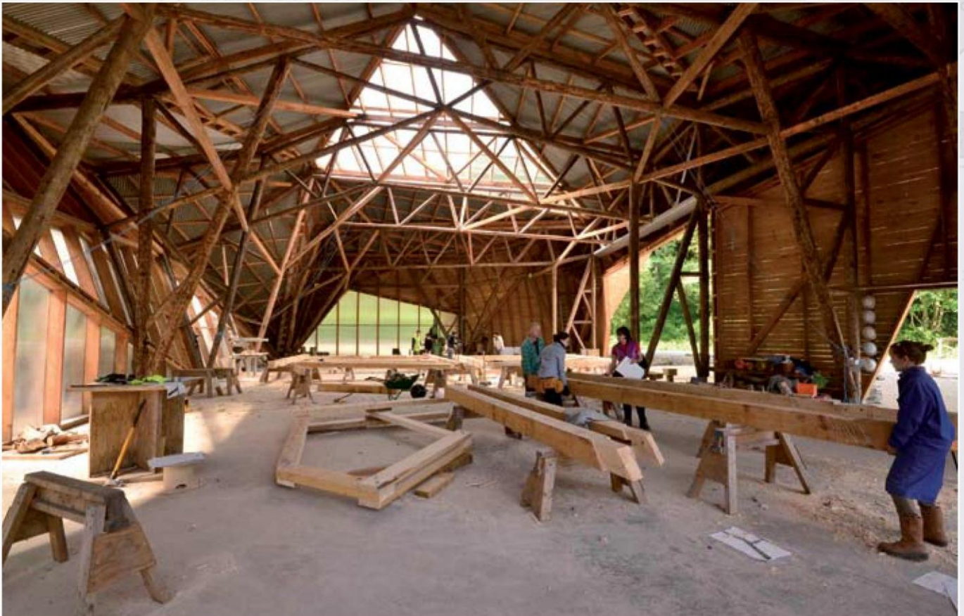
Interior view of the Big Shed
